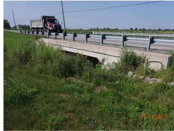
Photograph No. 2: 0248: East elevation.
