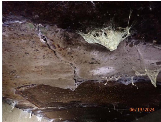
Photograph No. 4: 0449: Area of failure in concrete arch at west end of structure.
