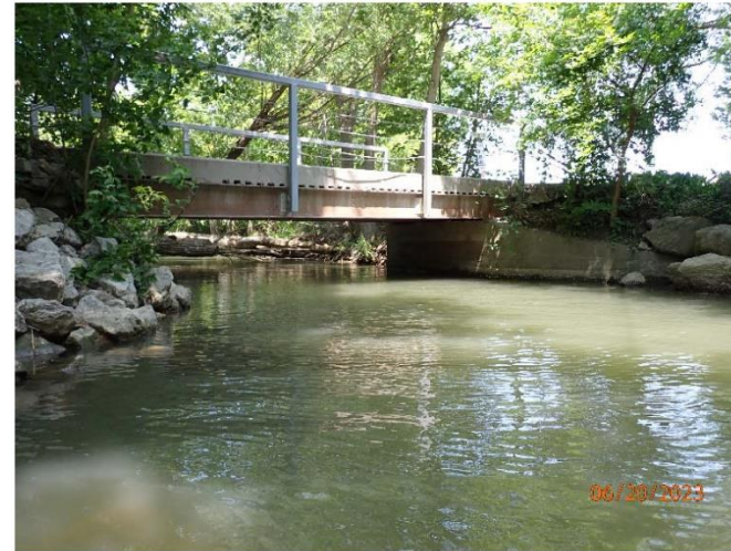
Photograph No. 2: 0771: South elevation.
