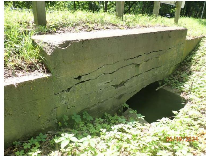
Photograph No. 2: 0437: West elevation.
