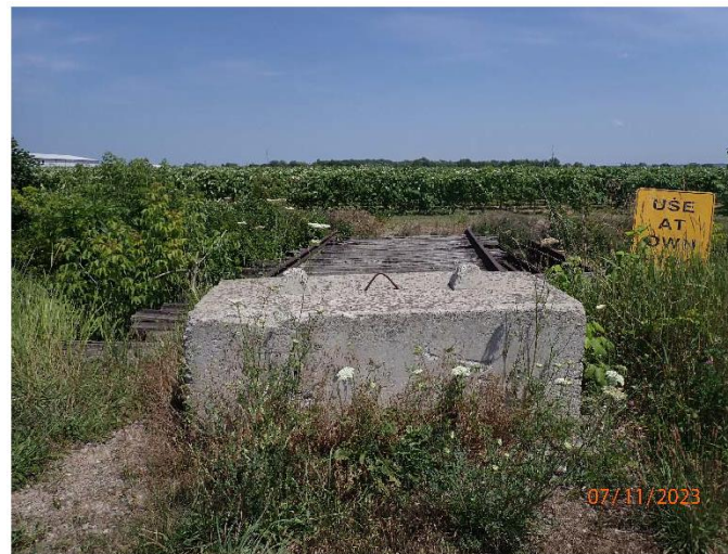
Photograph No. 4: 0722: Concrete barrier at west end.
