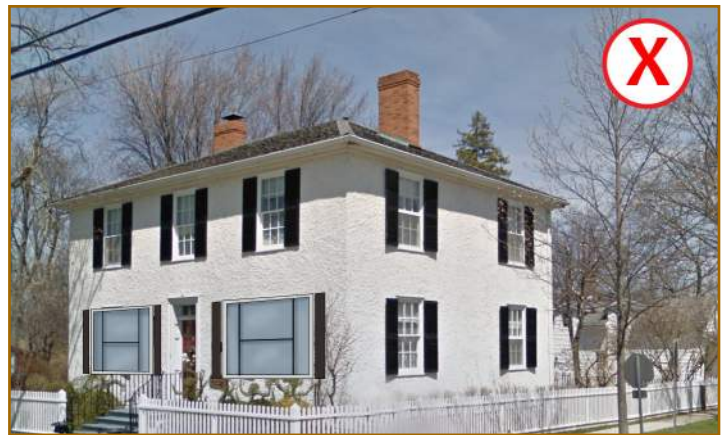
Figure 30 — Example of a incompatible alteration to a contributing property: replacement of front windows with a different size, form and materials.
