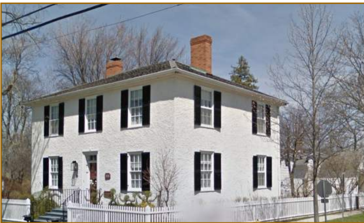
Figure 30 — Example of a incompatible alteration to a contributing property: replacement of front windows with a different size, form and materials.
