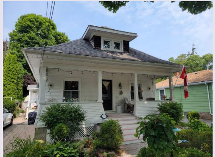
Figure 20 — Example of Edwardian architectural style, 133 Regent Street (Town of NOTL, 2025)
