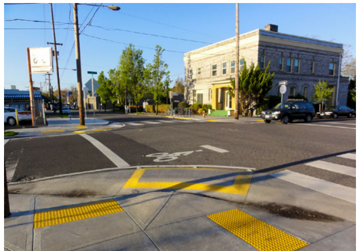
Flat mountable curb for bump out on a truck route (image: NACTO, CC BY-NC 2.0, Flickr)
