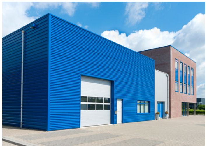
Colour, material and massing create a dynamic façade
