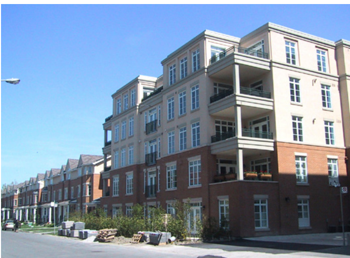
5 storey residential building with material palette matching adjacent low-rise residential uses
