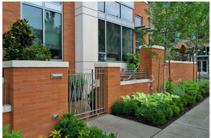
Raised terrace providing a transition zone between sidewalk and individual residential units
