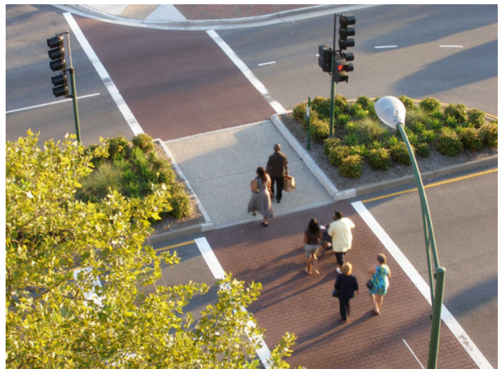
Pedestrian crosswalk defined by special paving and a refuge
