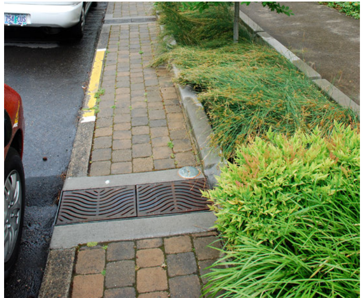
Bioretention planters for stormwater management, Portland OR
