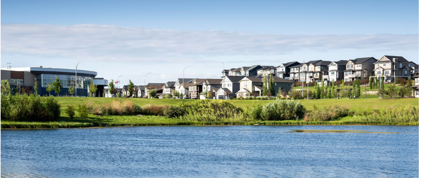
Stormwater pond integrated with school and recreational park uses
