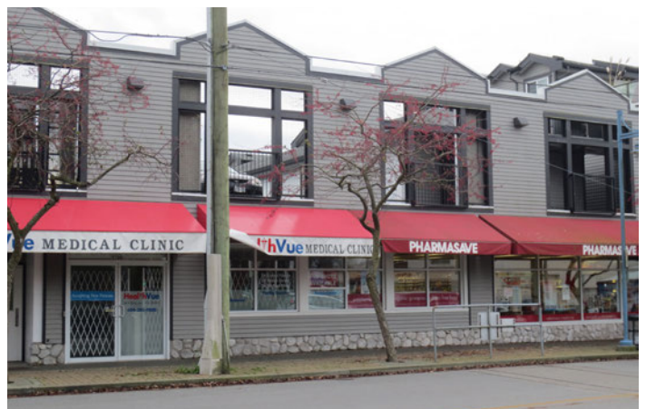
Parking structure with retail uses facing street at ground level
