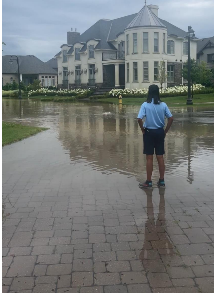
Figure 1. Photo of Flooding adjacent to stormwater management pond on July 10 th , 2024.
