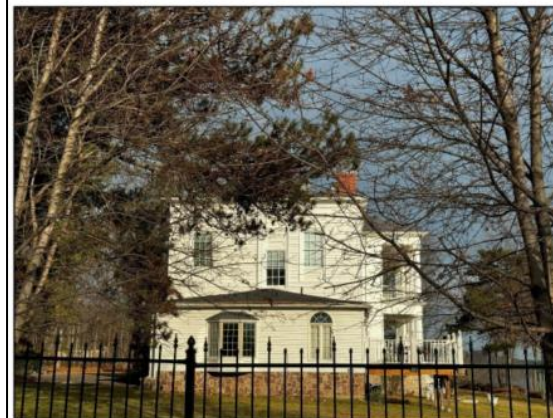
Image 2: South Elevation of Glencairn Hall (Image taken on: December 14, 2023)
