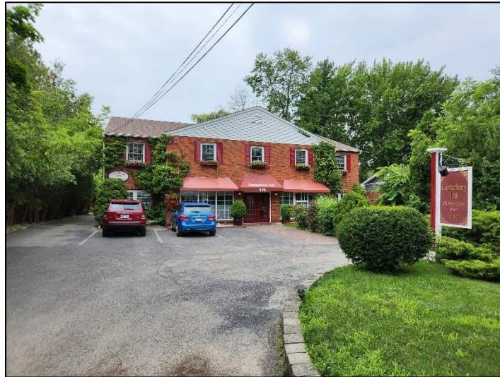
Figure 9 - 170 Mary Street - Canterbury Inn
