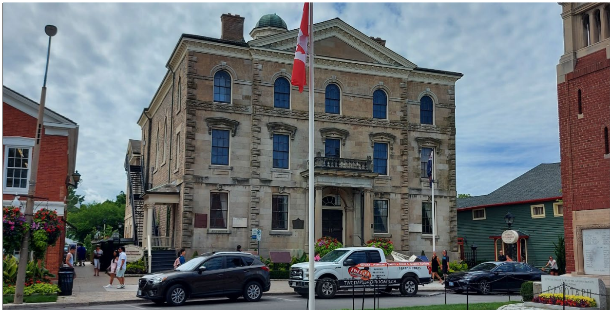
Figure 7: Old Niagara District courthouse
