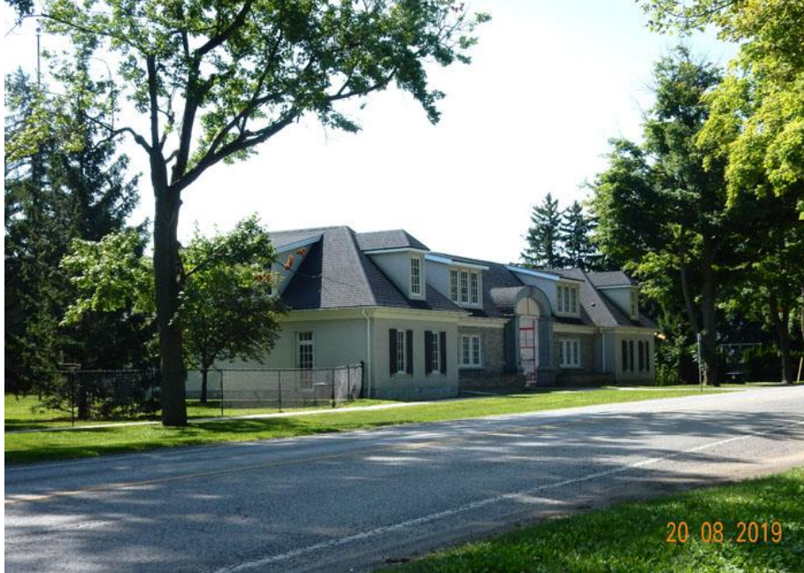
Figure 60: Mississagua Street East Side Looking Southeast, LDW
