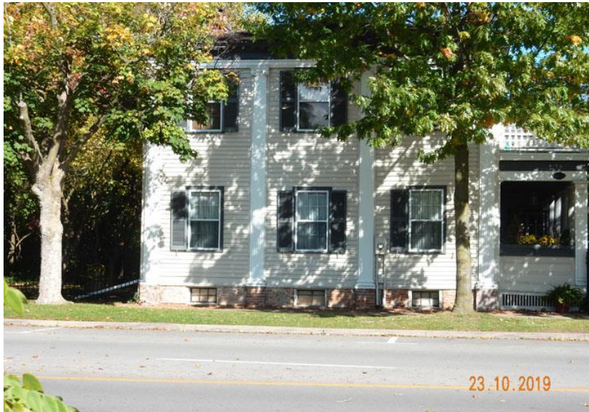
Figure 42: 187 Queen Street, Facade, LDW
