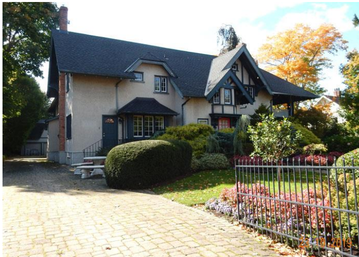
Figure 49: 164 Queen Street, Facade, LDW
