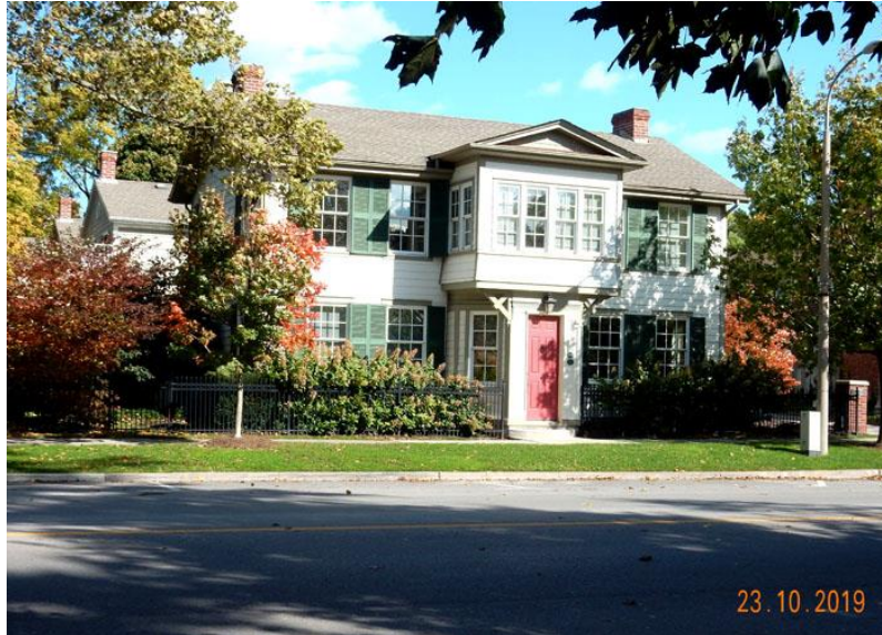
Figure 43: 175 Queen Street, Facade, LDW
