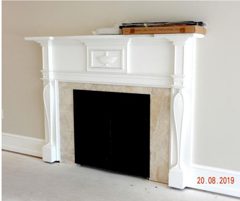
Figure 35: 228 Queen Street, Neo-classical Mantel, Main Floor, LDW
