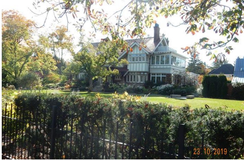
Figure 50: 184 Queen Street, Facade, LDW
