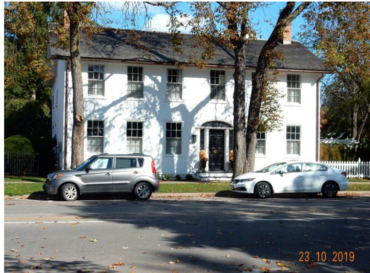
Figure 45: 157 Queen Street, Facade, LDW
