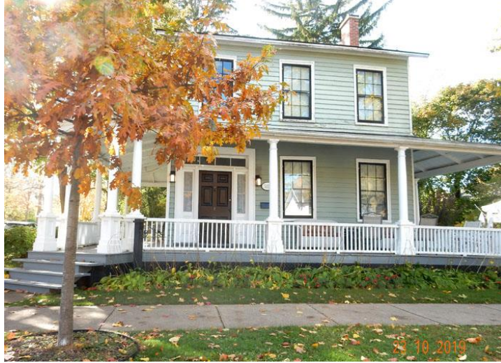
Figure 48: 154 Queen Street, Facade, LDW
