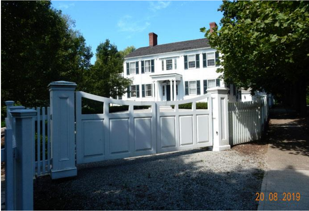
Figure 75 : Clench House, 234 Johnson Street Looking Southwest from Johnson Street
