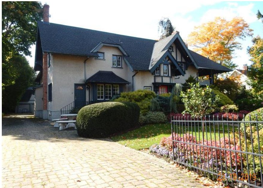
Figure 49: 164 Queen Street, Facade, LDW
