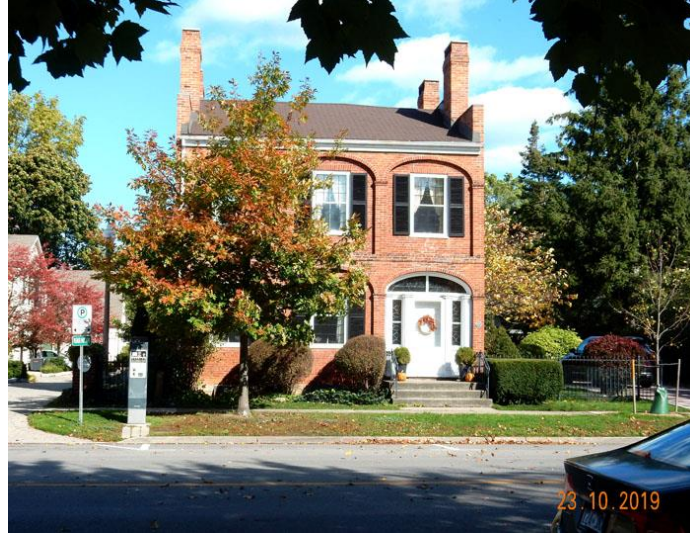
Figure 44: 165 Queen Street, Facade, LDW
