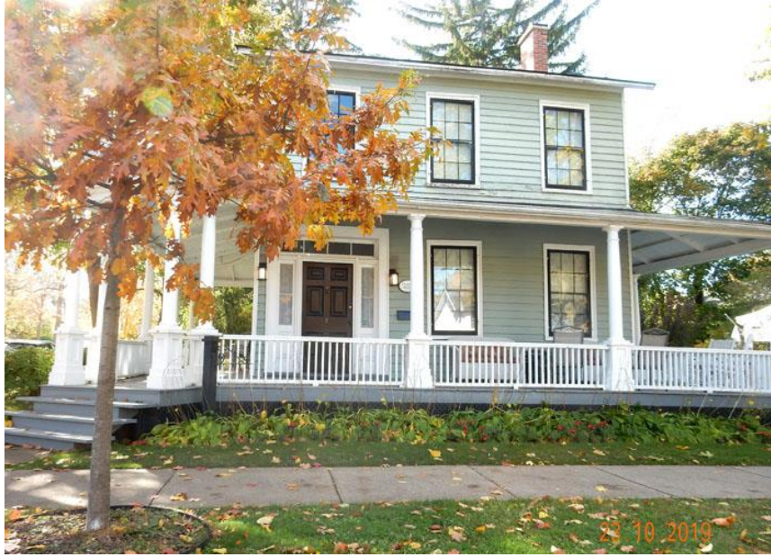
Figure 348: 154 Queen Street, Facade, LDW
