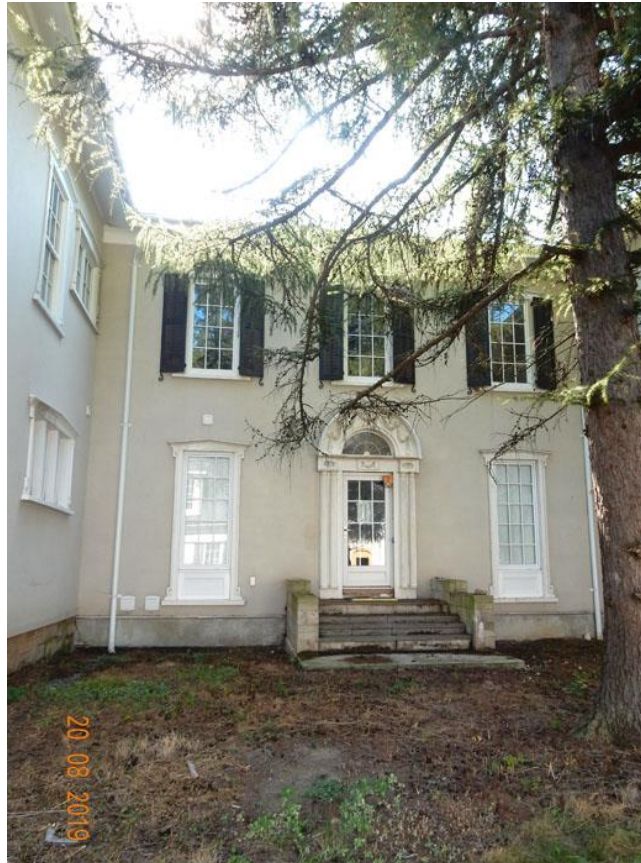
Figure 34: West Elevation, Rear Ell, Entrance Door, LDW
