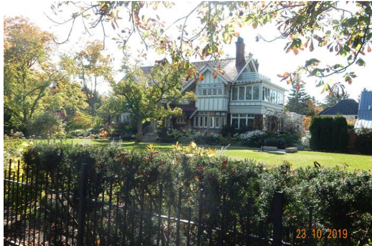
Figure 50: 184 Queen Street, Facade, LDW
