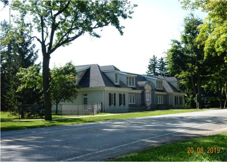
Figure 60: Mississagua Street East Side Looking Southeast, LDW
