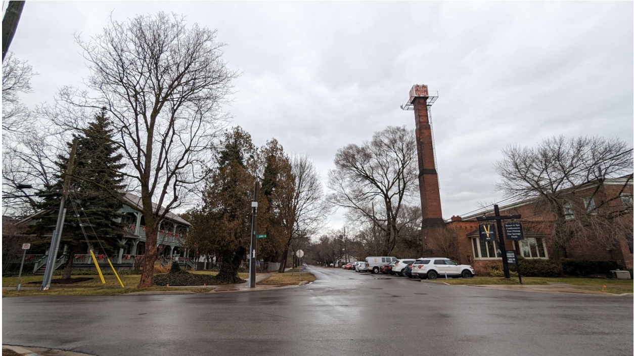
Photo 11: Pillar and Post
