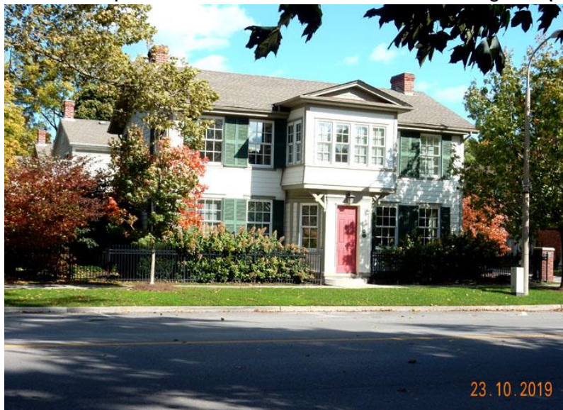
Figure 213: 175 Queen Street, Facade, LDW
