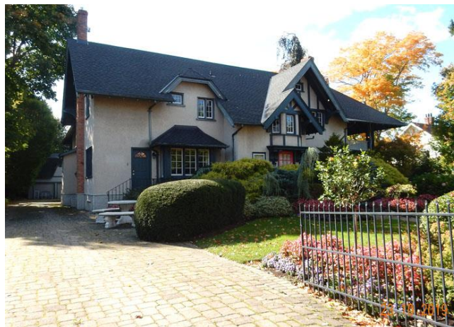
Figure29: 164 Queen Street, Facade, LDW
