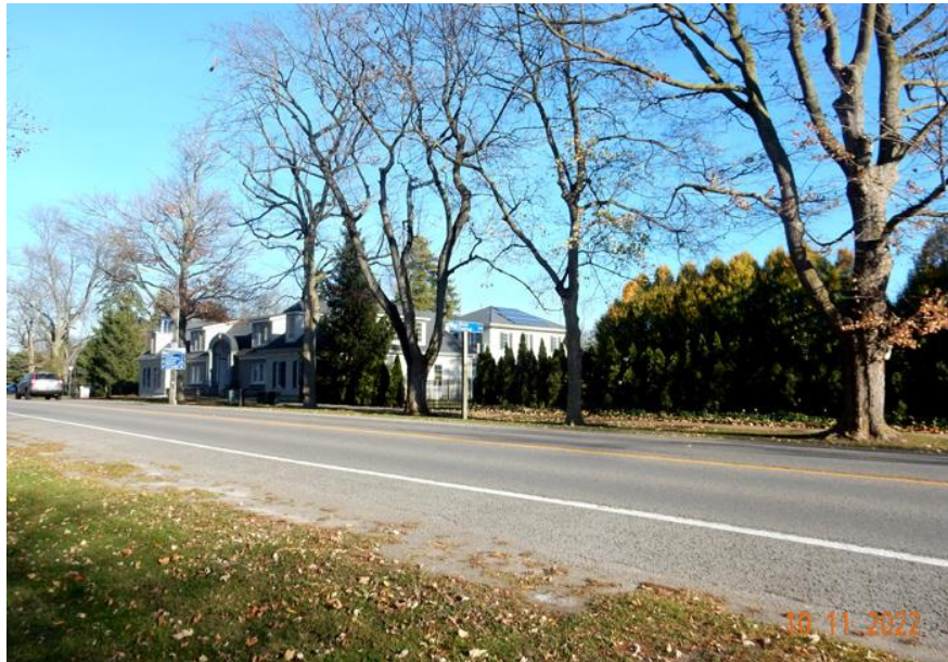
Figure 35: Mississagua Street Looking Northwest, 241 Johnson in Foreground, Newer Coach House & Peaceacres Upper Floor and Hip Roof in Background, LDW
