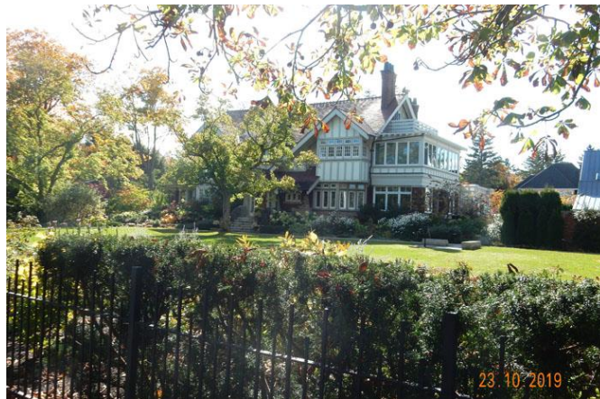
Figure 30: 184 Queen Street, Facade, LDW
