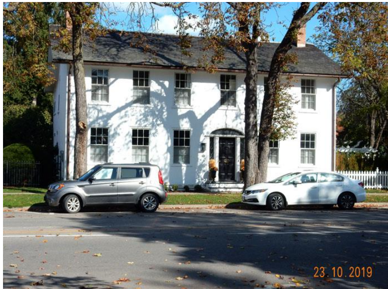
Figure 235: 157 Queen Street, Facade, LDW
