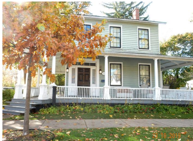
Figure 28 : 154 Queen Street, Facade, LDW
