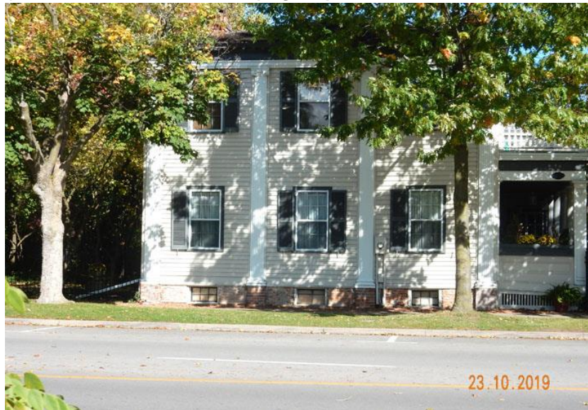
Figure 202: 187 Queen Street, Facade, LDW
