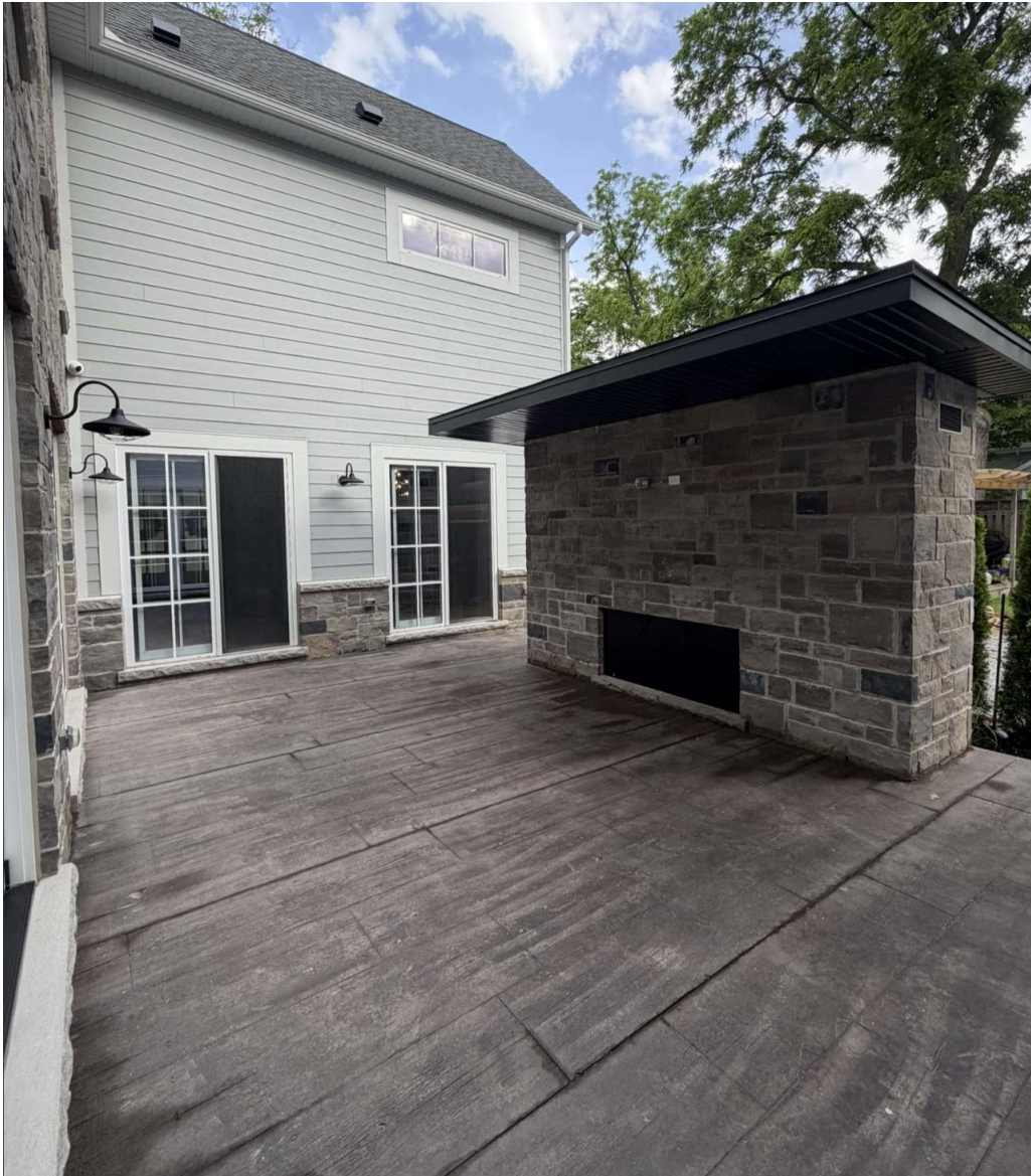
Photo 2. View of proposed location of lanai, inclusive of existing screening wall, from within building footprint.
