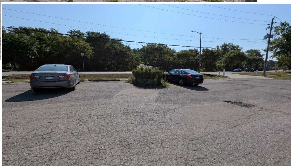
Photograph 24: This view is of Four Mile Creek Road showing the ditch and culverts for northern Site access. Photograph 25: This view shows the other Site access at the southern end of the Site.
