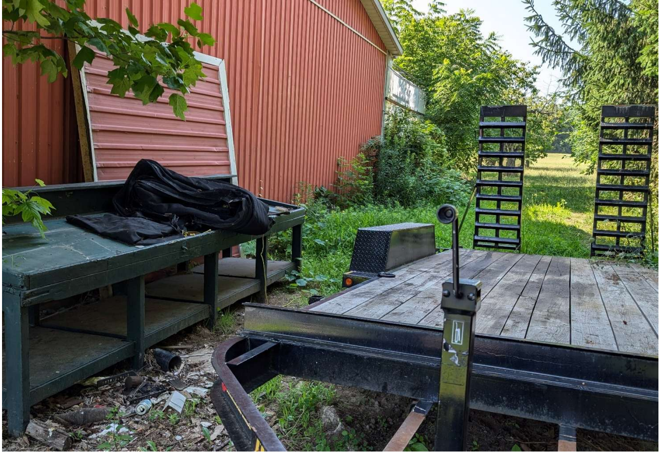
Photograph 2: This view is the rear of the building (west side) looking south along the western boundary of the Site. Note the small remnants of debris at the corner of the building.
