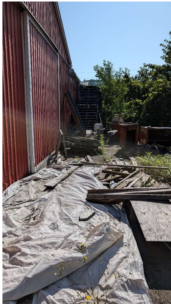
Photograph 4: Remnants of the greenhouse-like addition along the south side of the building.
