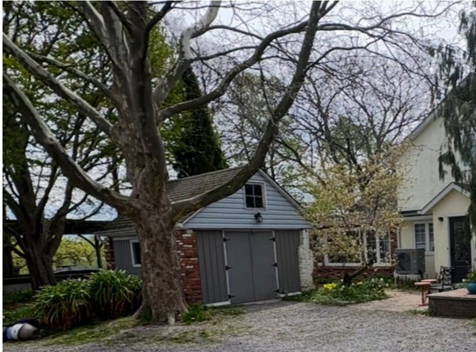
FIGURE 8: “Garage #1” as Identified on Surveyor’s Sketch (Appendix 1)
