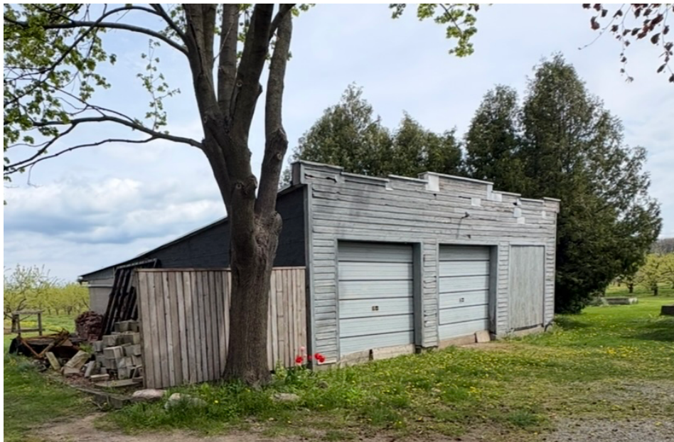
FIGURE 9: “Garage #2” as Identified on Surveyor’s Sketch (Appendix 1)
