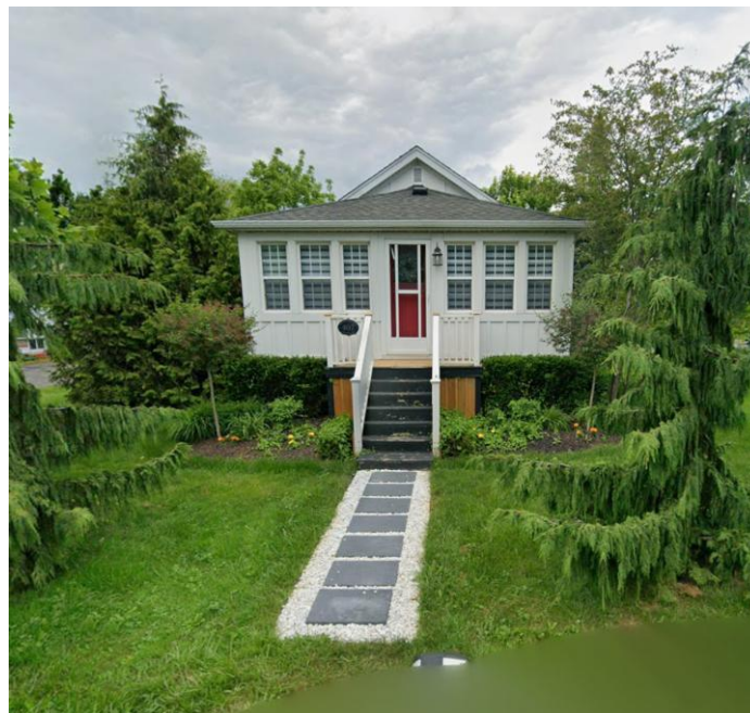
Photo 8. Google Streetview image of 407 Gate Street, located at the intersection of Gate Street and William Street (Source: Google Streetview, 2025)
