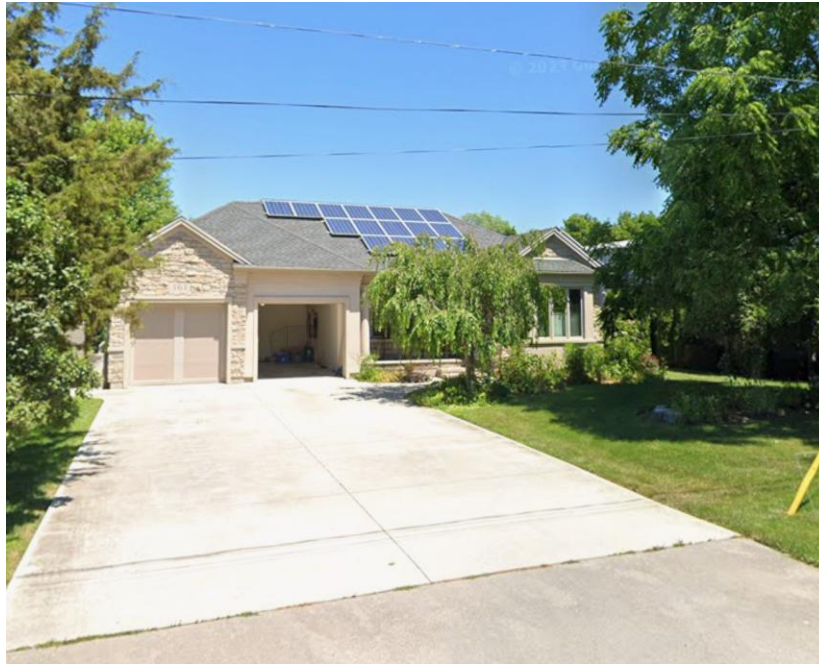
Photo 7. Google Streetview image of 161 William Street. (Source: Google Streetview, 2023)
