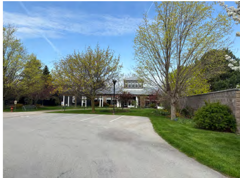
Photo B: View of Existing Entrance to Retail Store and Restaurant
