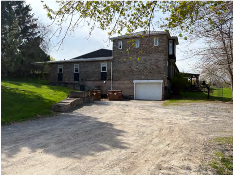
Photo E: View of Existing Service Entrance and Existing 2- storey Building (view from Lakeshore Road)
