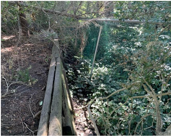
Photo 7 – Debris, both natural and manmade, exists at high densities throughout the reach.
