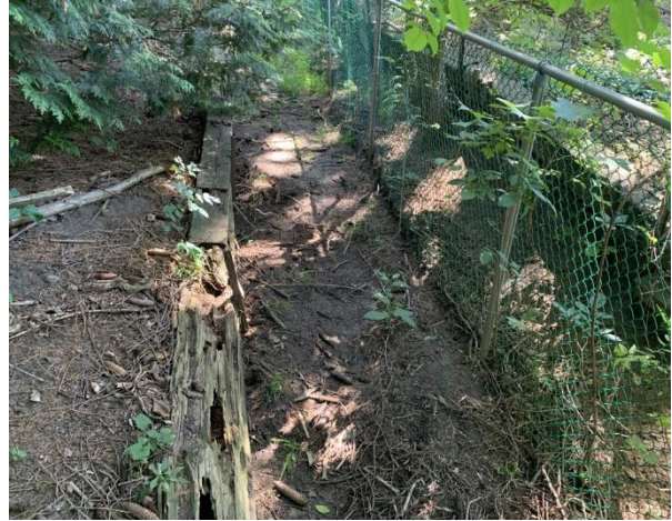
Photo 6 – Reach 2 presents as a heavily altered drainage feature, reinforced with revetments.
