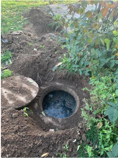
Septic Tank – Primary Chamber
