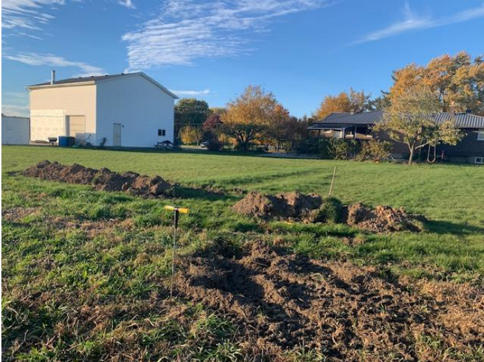
Trench Location – North Facing
