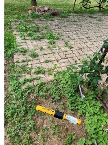
Septic Tank Probed
