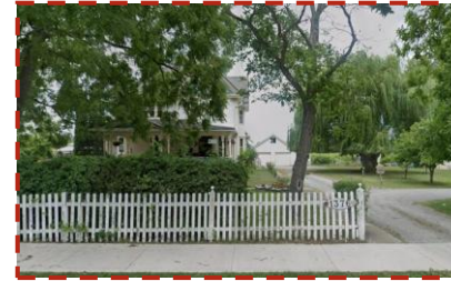
1376 YORK ROAD – EDWARDIAN STYLE (LISTED, NON-DESIGNATED HERITAGE PROPERTY ON THE TOWN'S HERITAGE REGISTER)
