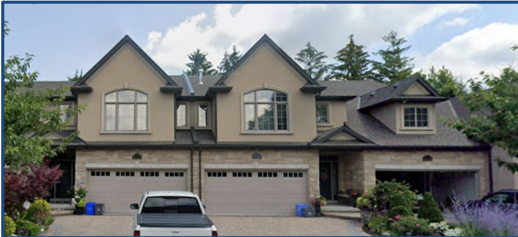
Figure 11 – Study Area 4- 607 King Street - Google Street View – July 2023
