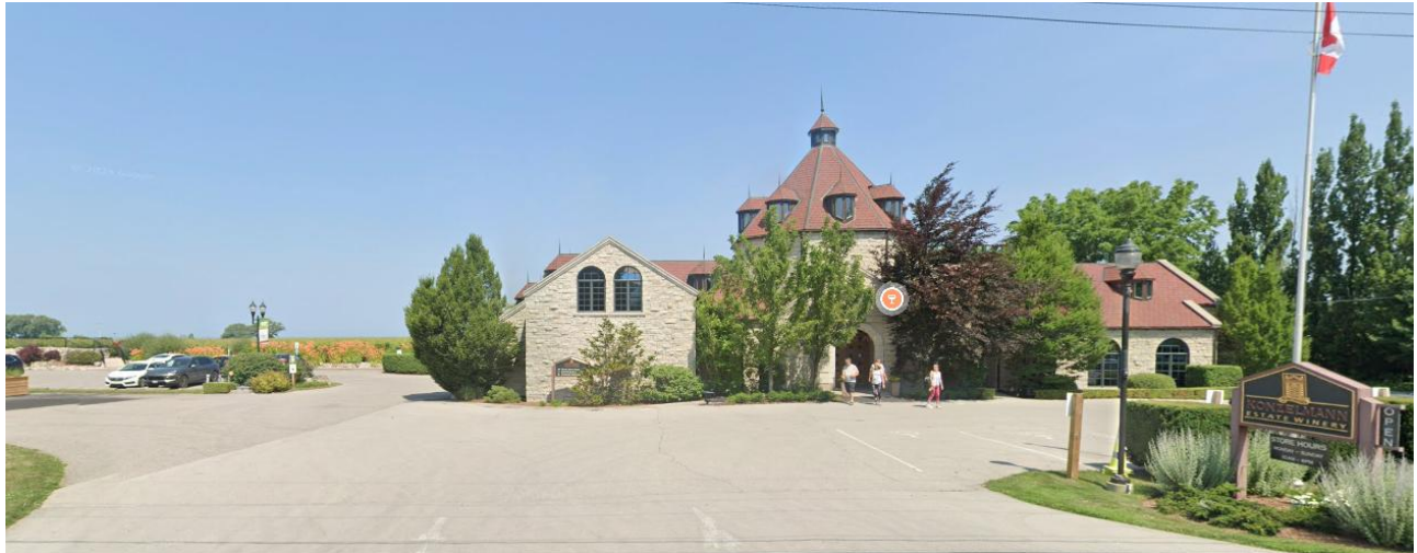
FIGURE 3: STREET VIEW OF SUBJECT LANDS (GOOGLE MAPS)
