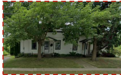
1367 YORK ROAD – FLOOR BEAMS AND HAND-Hewn LOGS (LISTED, NON-DESIGNATED HERITAGE PROPERTY ON THE TOWN'S HERITAGE REGISTER)
