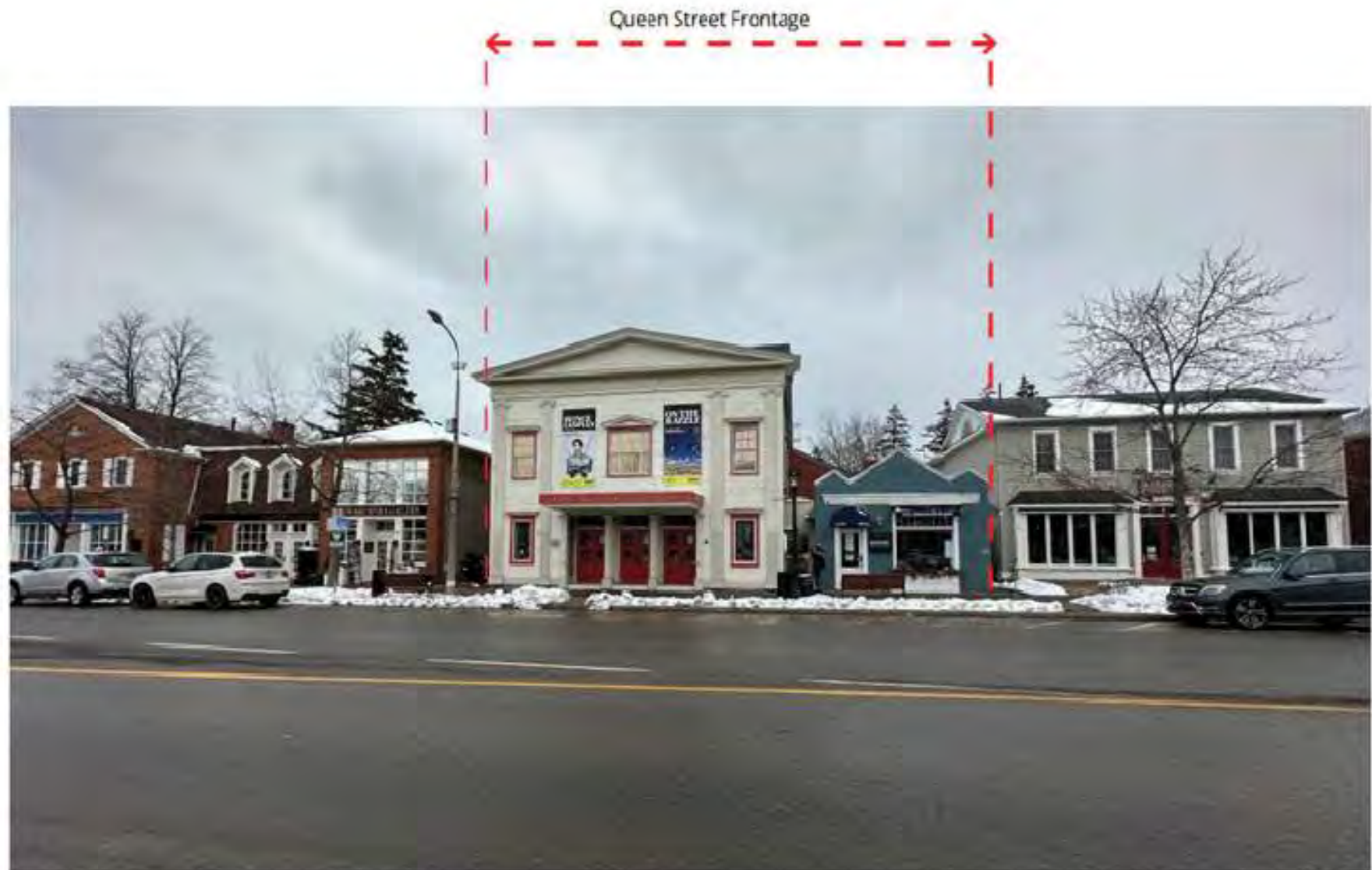
FIGURE 5. VIEW OF THE ROYAL GEORGE THEATRE AND ADJACENT PROPERTIES ALONG THE QUEEN STREET FRONTAGE, ILLUSTRATING THE CONTINUOUS LOW-RISE BUILT FORM, PEDESTRIAN SCALE, AND COHESIVE STREETScape CHARACTER WITHIN THE QUEEN-PICTON HERITAGE CONSERVATION DISTRICT. SOURCE: MCCALLUMSATHER, 2023.
