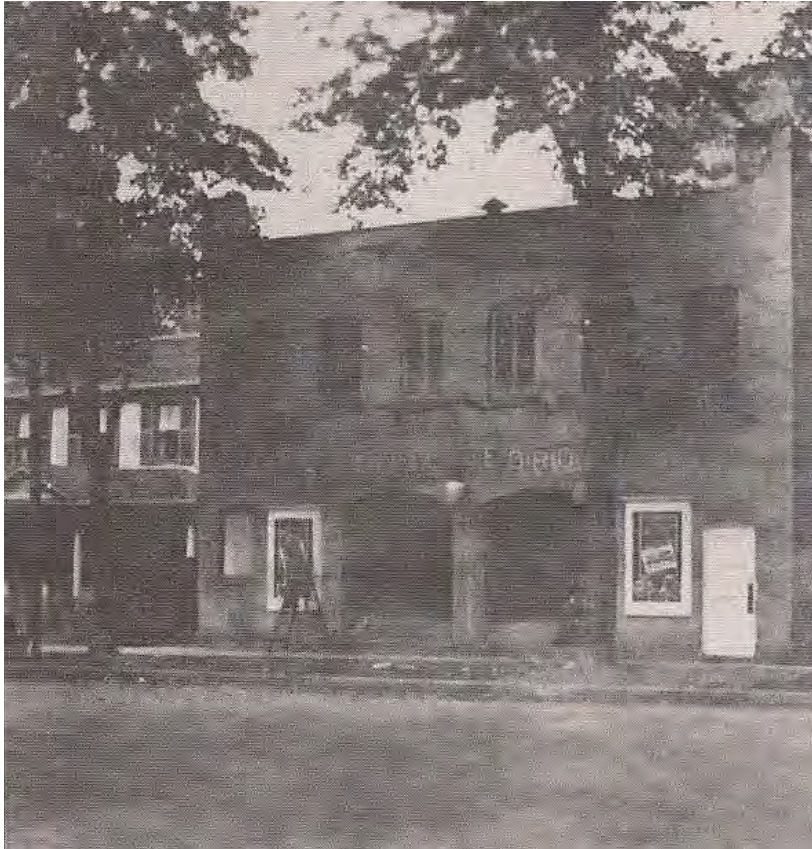
FIGURE 11. THEATRE UNDER OWNERSHIP OF GEORGE REID, WHO RENAMED A QUEEN STREET VENUE THE ROYAL GEORGE. NOTE: THIS MAY DEPICT THE EARLIER ROYAL GEORGE THEATRE, A SEPARATE STRUCTURE DEMOLISHED IN THE 1930S. SOURCE: "LOOKING BACK: NIAGARA-ON-THE-LAKE, ONTARIO" BY CLARK BERNAT AND JOY ORMSBY (2003). PHOTO COURTESY OF MRS. PATRICIA MCCARTHY, AS PUBLISHED IN THE REFERENCED WORK.
