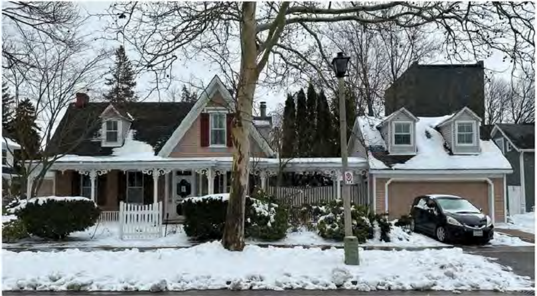
FIGURE 10. VIEW OF 178 VICTORIA STREET, SHOWING THE TWO-STOREY RESIDENTIAL BUILDING AND ASSOCIATED GARAGE. THE PROPERTY CONTRIBUTES TO THE MIXED RESIDENTIAL CHARACTER OF VICTORIA STREET WITHIN THE QUEEN-PICTON HERITAGE CONSERVATION DISTRICT. SOURCE: MCCALLUMSATHER, 2023.
