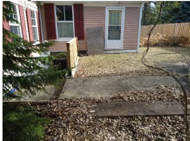
Plate 10: View of walkway and entrance to basement.
