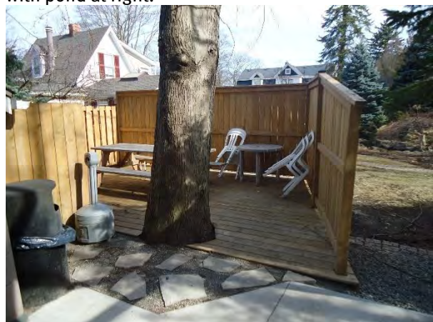
Plate 6: Wooden deck connected to walkway behind theatre.
