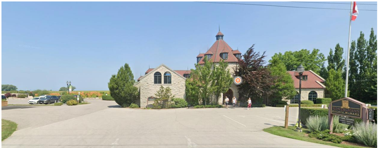
FIGURE 3: STREET VIEW OF SUBJECT LANDS (GOOGLE MAPS)
