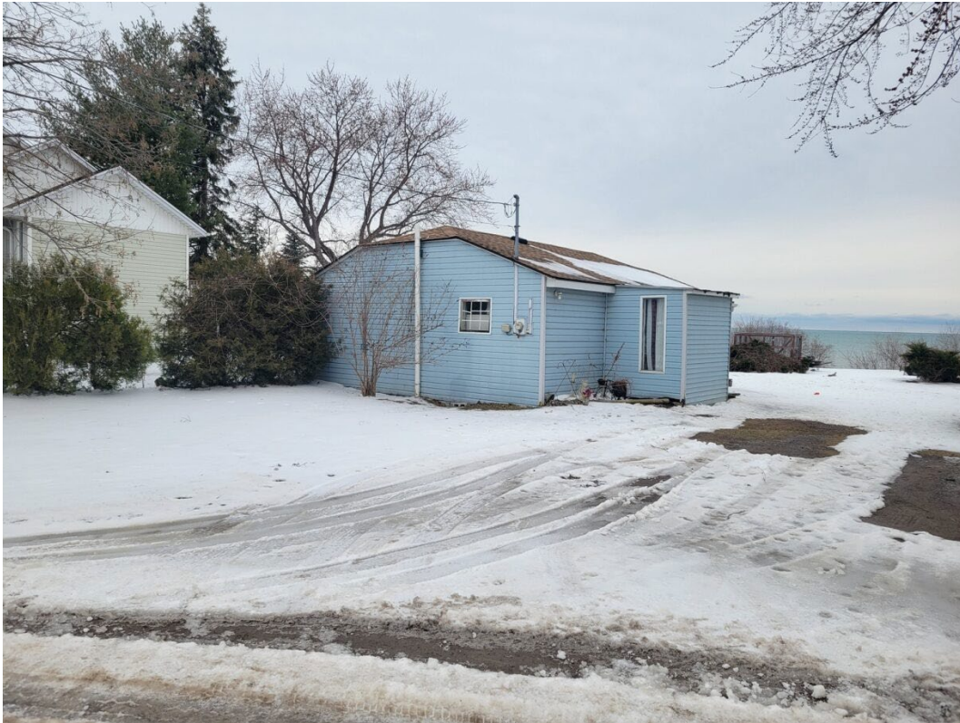
Photo 3. View looking north towards 4 Firelane 13B.
