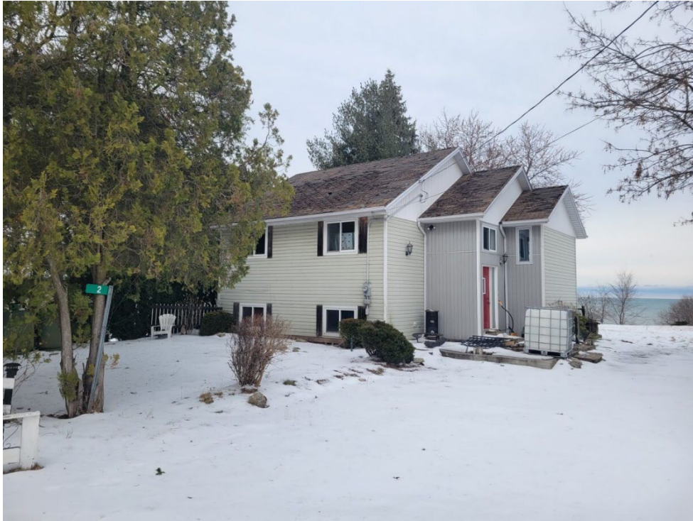
Photo 1. View looking north towards 2 Firelane 13B.
