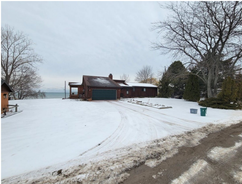
Photo 8. Looking north towards 10 Firelane 13B.
