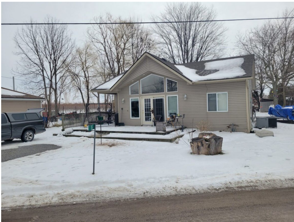
Photo 4. View looking south towards 5 Firelane 13B. Note this property is not part of the application.
