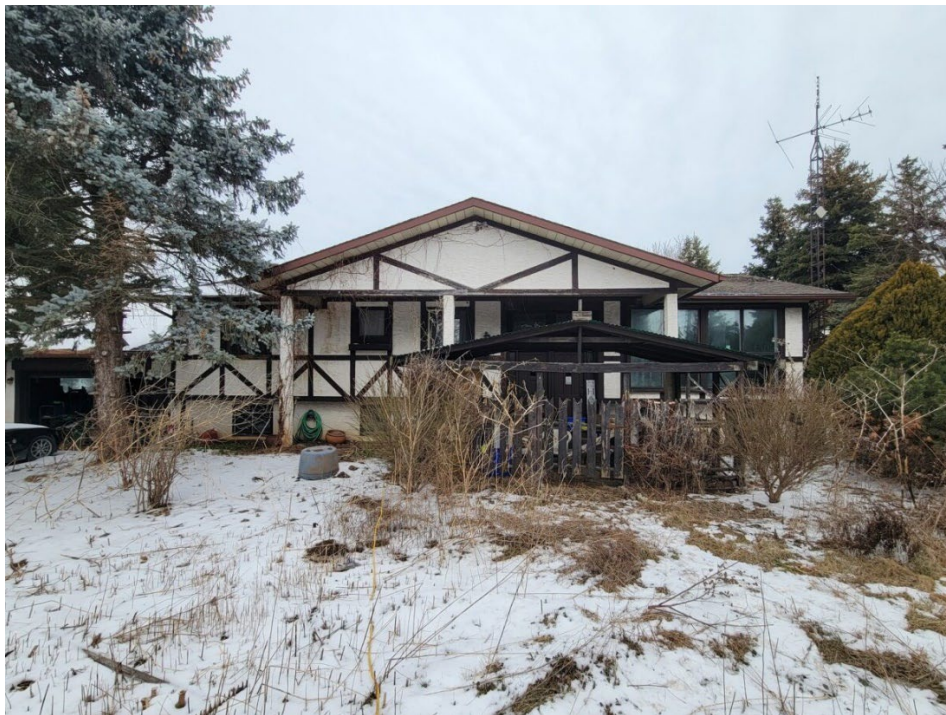
Photo 10. Looking north towards 14 Firelane 13B.
