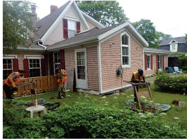
Plate 2: Test pit survey in progress at rear of 178 Victoria Street.
