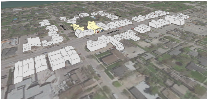
Existing Aerial View
