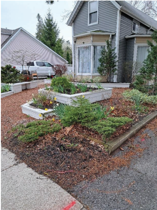
Image 1: View of the southwest corner and front of the house at 188 Victoria Street.
