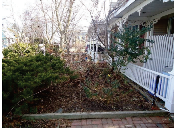
Plate 8: Front garden with blue and yellow flags marking buried utilities.
