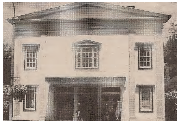
FIGURE 14. ROYAL GEORGE THEATRE AFTER THE 1980S RENOVATION—GEORGIAN-REVIVAL FACADE WITH SMOOTH STUCCO, CORNER PILASTERS, HIGH PARAPET, AND CENTRED MULTI-PANE SASH WINDOWS REINSTATES CLASSICAL SYMMETRY ON QUEEN STREET.
