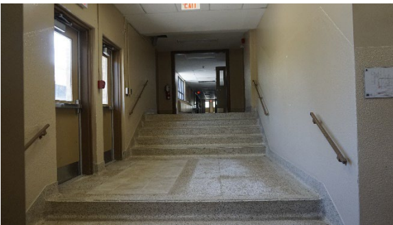
Photo 33: Terrazzo stairs between 1948 structure and 1953 addition
