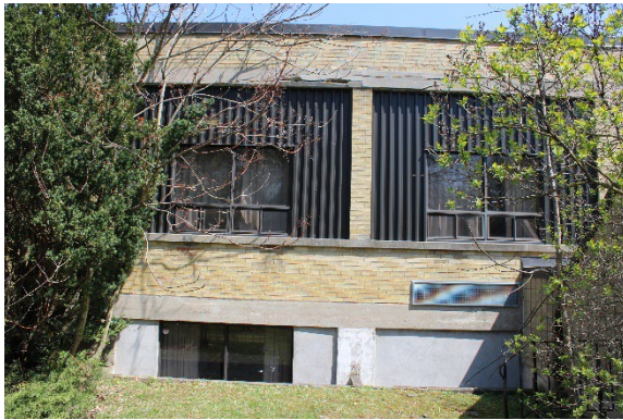
Photo 20: Typical windows and basement windows with egress stair on right
