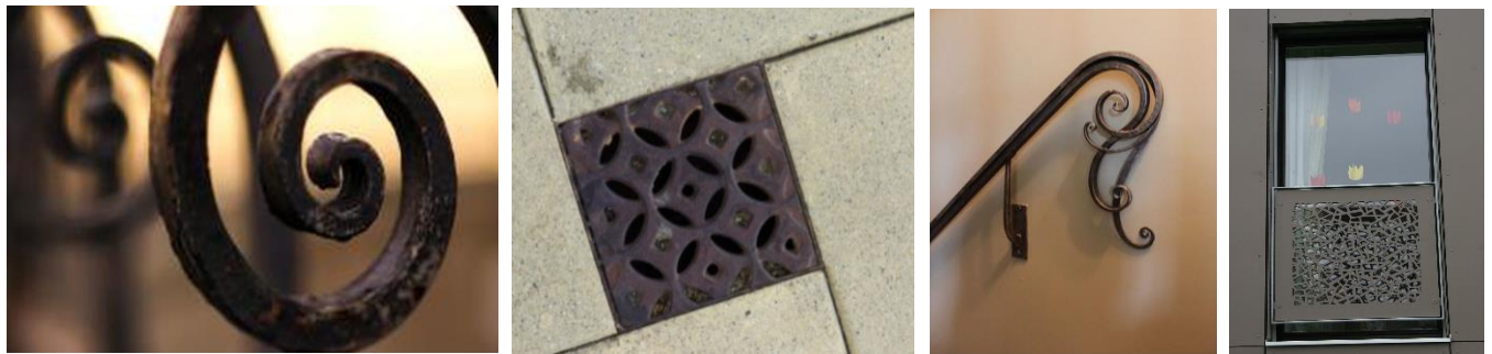
Figure 75- Collage: character/style examples of wrought iron and decorative metal grates/ wall panels over equipment vents, etc.
