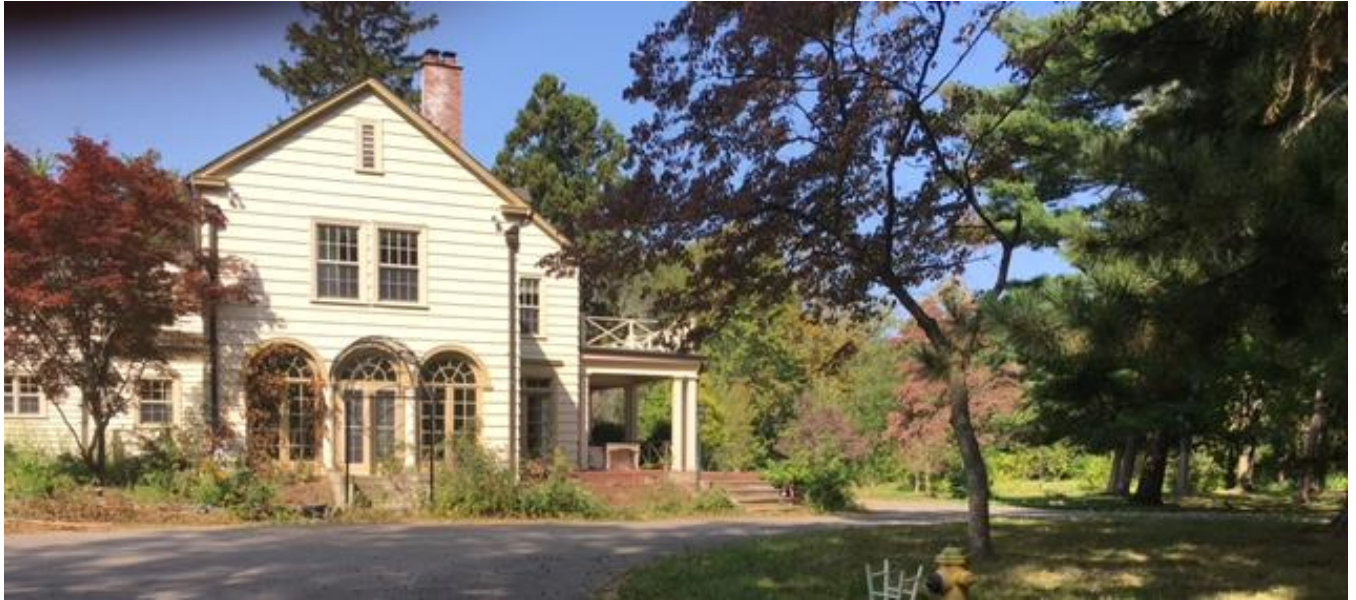
Figures 3, 4 & 5 - (above) Devonian House- east elevation; (below ) Coach House – north (Left) and west (right) elevations
