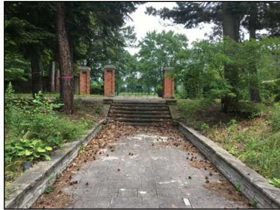
Entrance Gate (Central Access Point)
