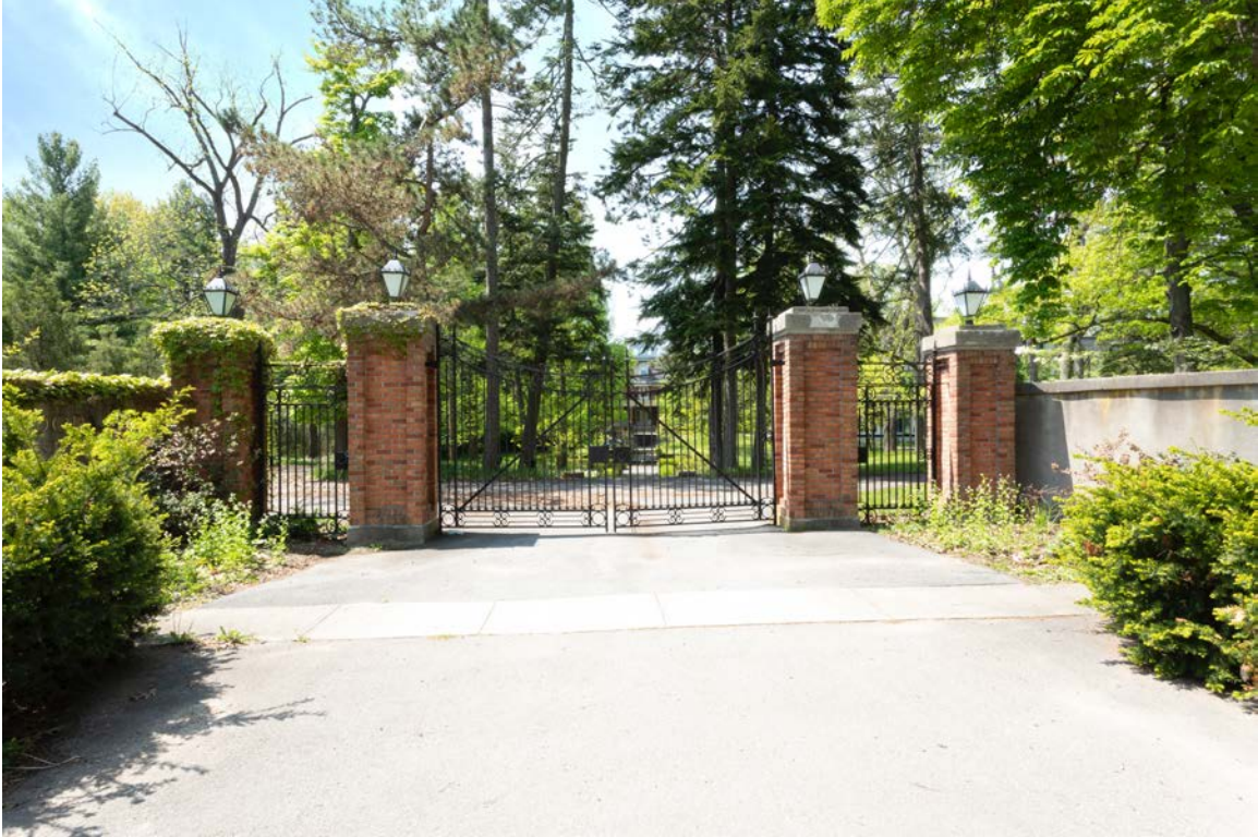
18A – View from John Street
